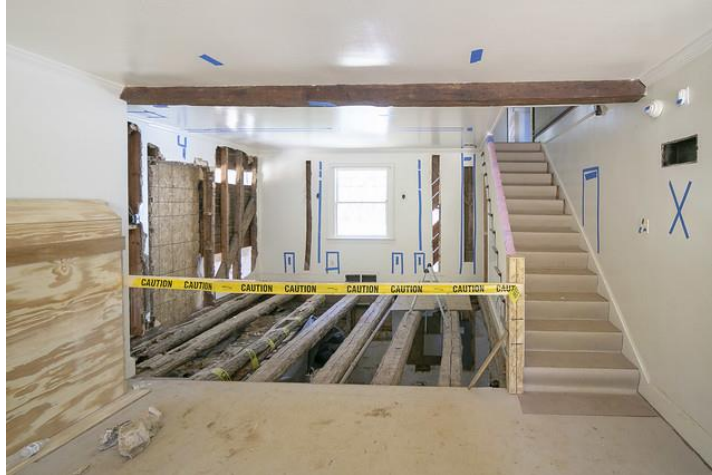
House interior during Museum construction (MCP)
