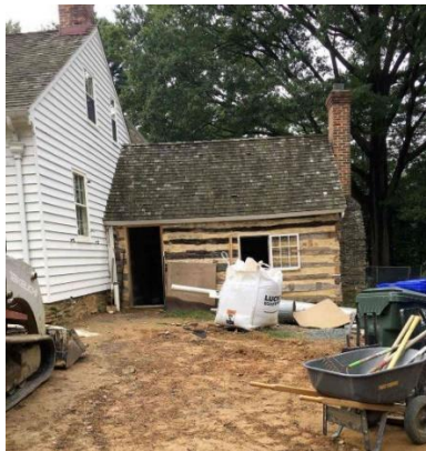
Henson slave cabin during Museum construction (LT)
