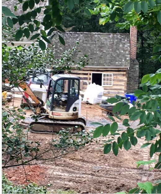
Henson slave cabin as seen from the street during construction (LT)
